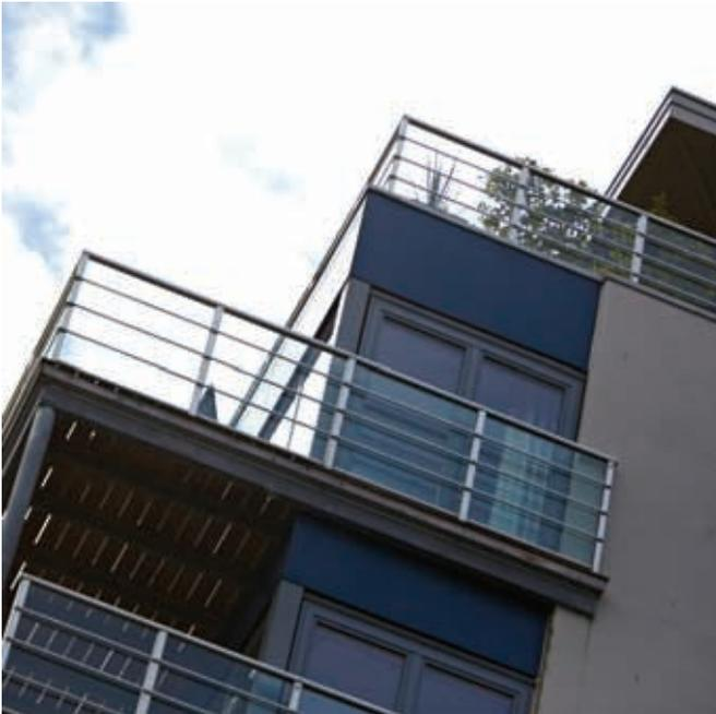
**Solution 1** Aesthetics mid-rails behind glass infill panels
